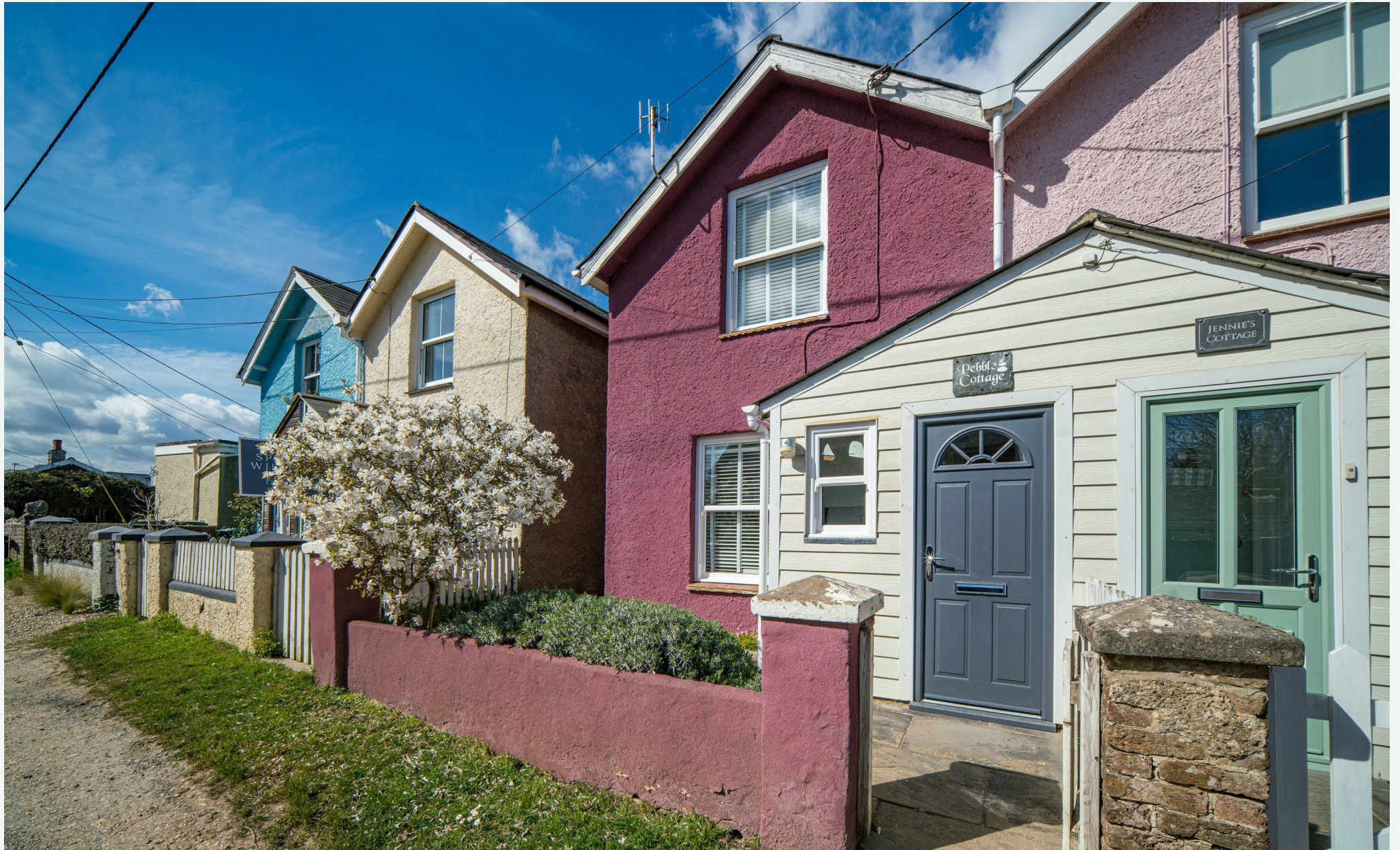
Pebble Cottage 6 Solent View, Queens Road, Bembridge, Isle Of Wight, PO35 5UT
